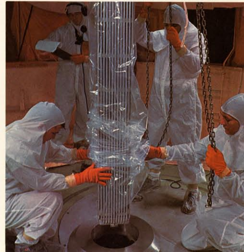
Technicians guide a reactor fuel element into position.
