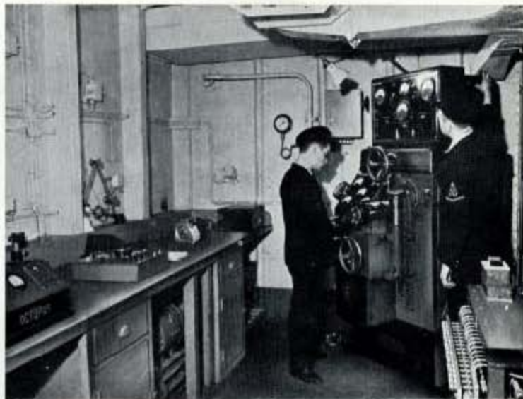
Fig. 352—A view in the Electrical Repair Shop on the gallery deck, showing an Octopus generator testing machine in use; on the bench is an Octopus armature drop tester and a bomb release test panel.
