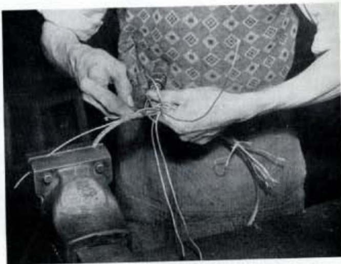
Fig. 292.—Splicing one of the securing straps which fits round the oleo leg of an aircraft for securing when ship borne.
