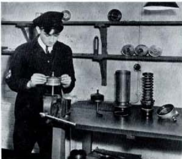
Fig. 216—The Engine Starter Repair Bay is another of the ancillary workshops. Here is a local modification being carried out to an Eclipse cartridge starter.
