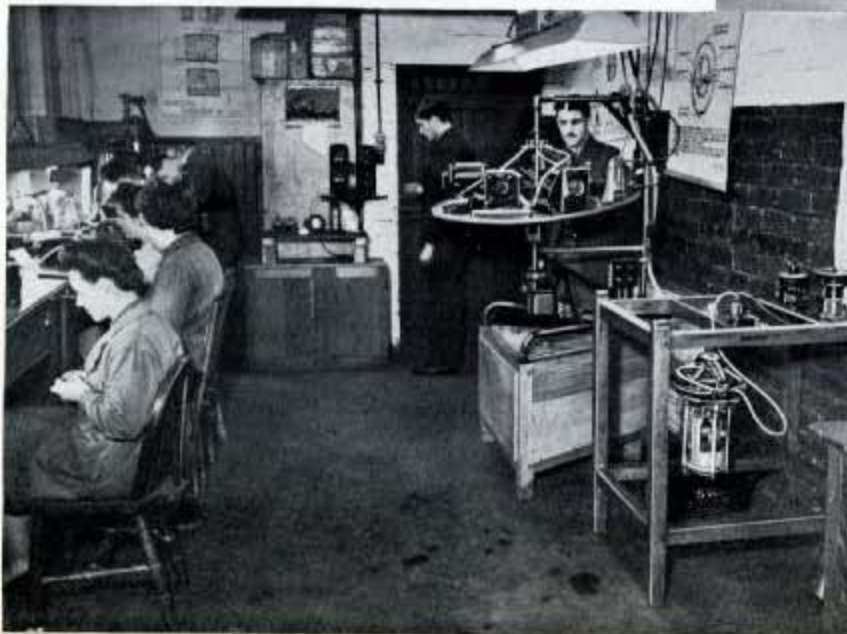
Fig. 257—A view in the Instrument Repair Shop which deals with the maintenance and test of altimeters, air speed and engine speed indicators, rates of climb indicators, oxygen equipment, etc.
