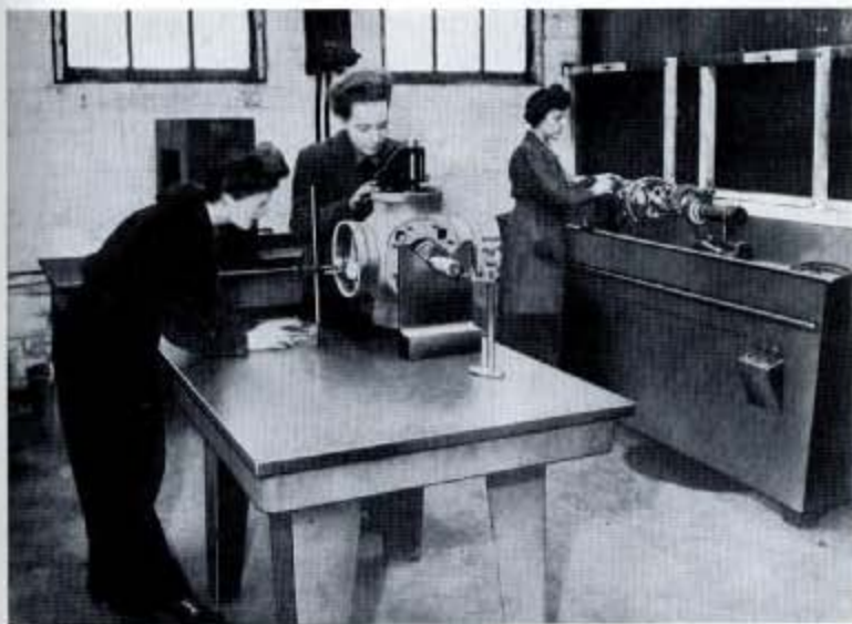
Fig. 226—In the Inspection and View Room; at the table the track of a Rotol propeller hub is being checked with a dial gauge; the other instrument being used for checking the divide of the ports. The inspector at the rear is examining components for cracks on the electric crack detector.
