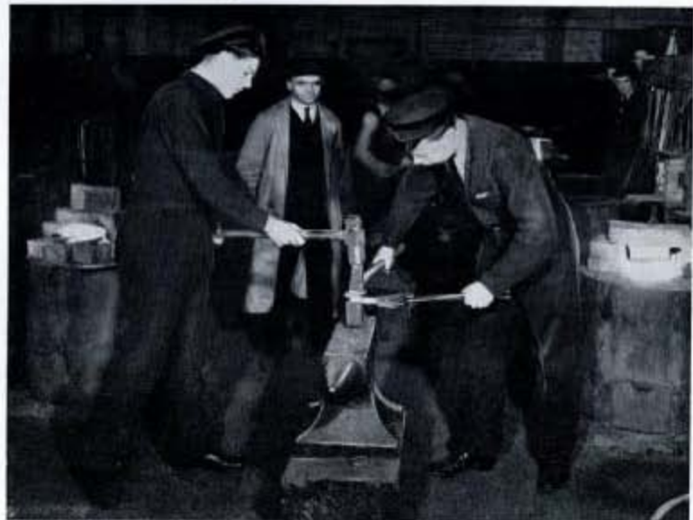
Fig. 34—Fitters and Turners (D Class, 1½ to 2 year period) forging a hexagon headed bolt as practice work during their 4 weeks Engin smithing Course.
