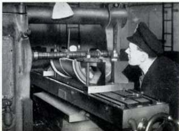
Fig. 151 (Below)—A bevel milling cutter set-up for machining the oil-way chamfer in one half of the main engine bearing shown being bored in Fig. 149.
