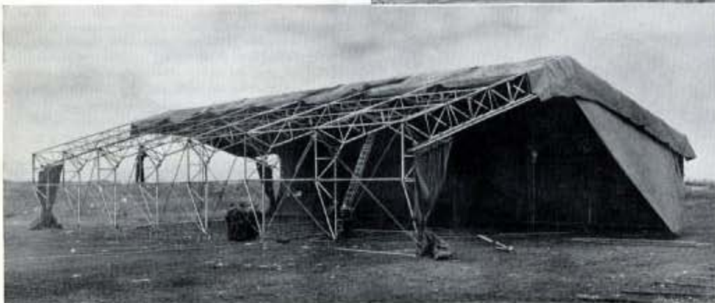
Fig. 333 (Above)—The tarpaulin end walls of the hangar are attached to runways with heavy roller type curtain fittings.
