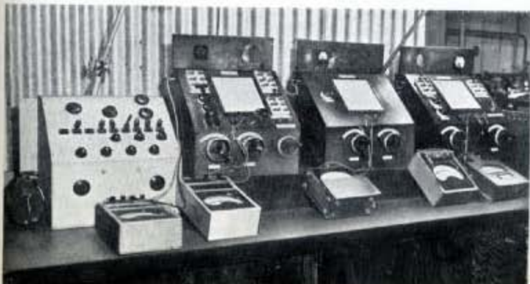
Fig. 300 (Left)—Meter test panels in the Electrical Shop; the meters under test should normally be flat and are only raised at an angle for the photograph.
