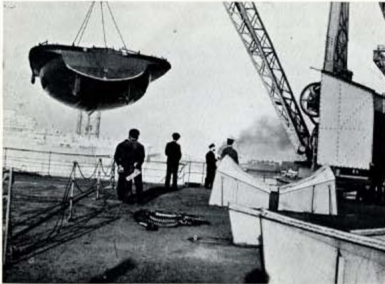
Fig. 348—From this angle one of the lighter cradles on the 'flight' deck is shown more clearly; in this view and in Fig. 347, the new aircraft carrier Implacable will be seen lying at anchor in the background.
