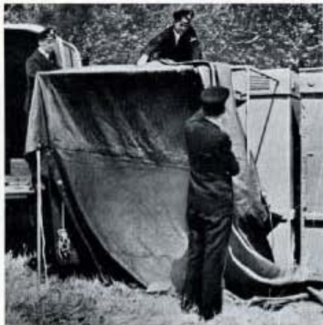
Fig. 325—Erecting the black-out entrance to one of the workshop stores of the M.A.R. Component. This enables night work to be carried out in the forward areas.
