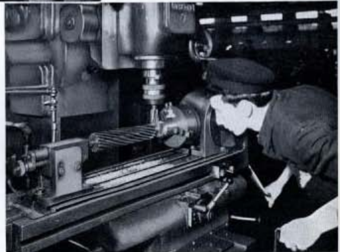
Fig. 41—F Class (2½ to 3 year period) Fitters and Turners and Electrical Artificers spend 2 weeks on milling practice; here a square is being milled on a helical toothed pinion.
