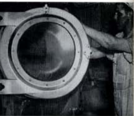
Fig. 161—The finished door fitted to the washing machine in the ship's laundry.
