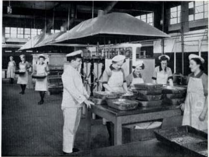
Fig. 84—A view in the Main Galley showing steam cookers in the foreground with domestic ovens in the rear.
