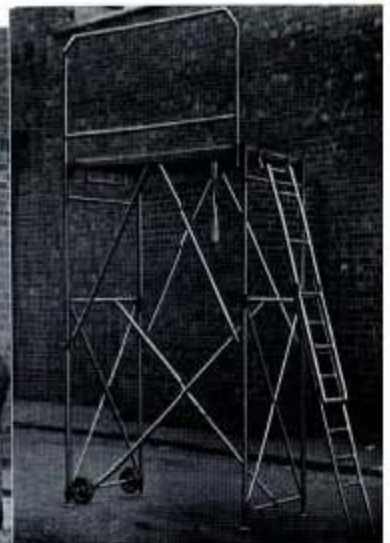
Fig. 213—The completed platform ready for use.
