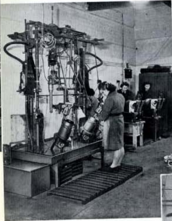
Fig. 249—The Valve and Valve Seat Section of the E.R.S. In the foreground is a special rig for Merlin and Pegasus cylinders; the two machines in the rear are Bristol valve seat grinders.
