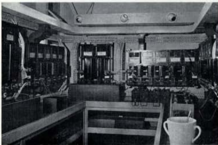
Fig. 353—This Battery Charging Room on the gallery deck has 26 panels, with meters, for aircraft batteries (including heavy duty type such as starter batteries) as well as those for use in the motor boats.
