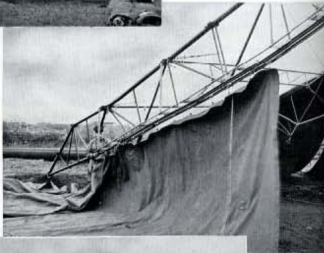
Fig. 333 (Above)—The tarpaulin end walls of the hangar are attached to runways with heavy roller type curtain fittings.
