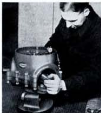
Fig. 233—To ensure correct balance, the concentricity of the Hamilton Hydromatic propeller hub must be within a maximum error of .004".
