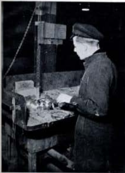
Fig. 36—In the D Class period, Fitters and Turners also spend 2 weeks in the Boiler Shop and 4 weeks Coppersmithing; practice work in the latter course is here depicted, the apprentice brazing flanges and unions to a copper pipe.
