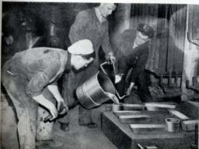
Fig. 158 (Left)—The next stage of pouring the aluminium into the mould for the new door.
