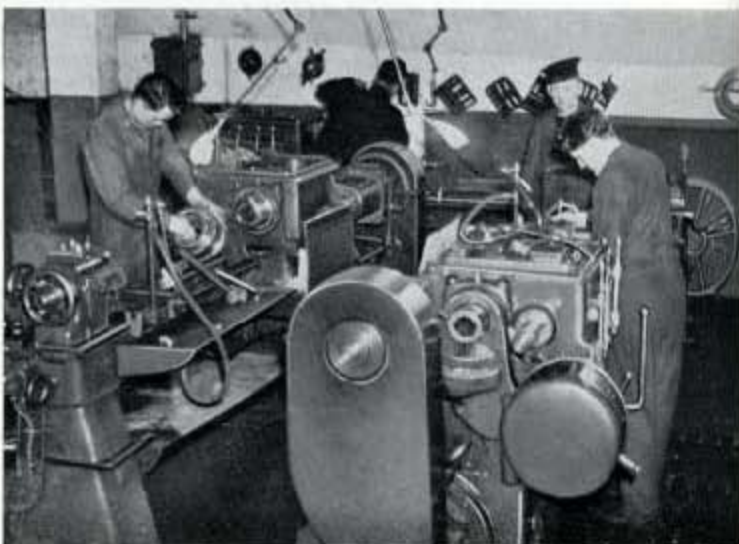
Fig. 144—A group of Lang lathes with all-g geared headstocks and individual motor drive in a corner of a Repair Ship Machine Shop.
