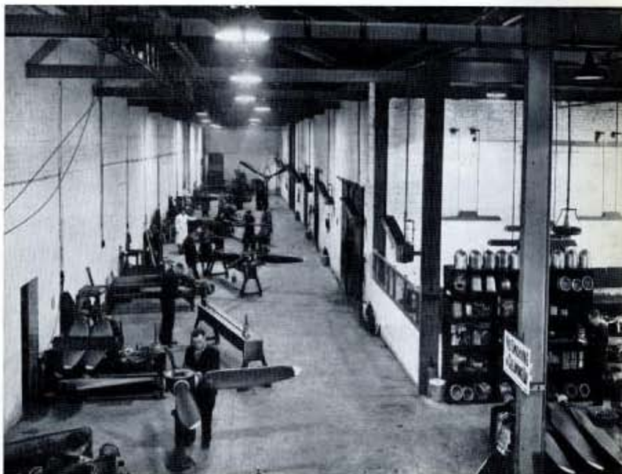
Fig. 225—One of the first components to be removed from the aircraft is the propeller, and this is sent to the Propeller Shop, an ancillary workshop at Dundee; here is a general view in the Assembly Bay.
